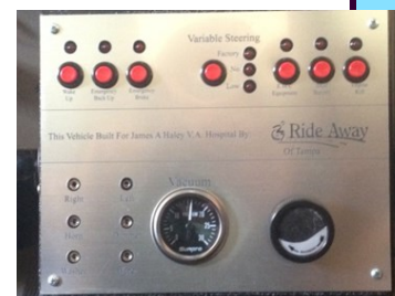
Switchboard: Custom made switchboard for secondary functions, variable effort steering and braking, emergency brake, emergency back-up, emergency kill switch, electronic gas/brake and steering activation, and back-up battery.
